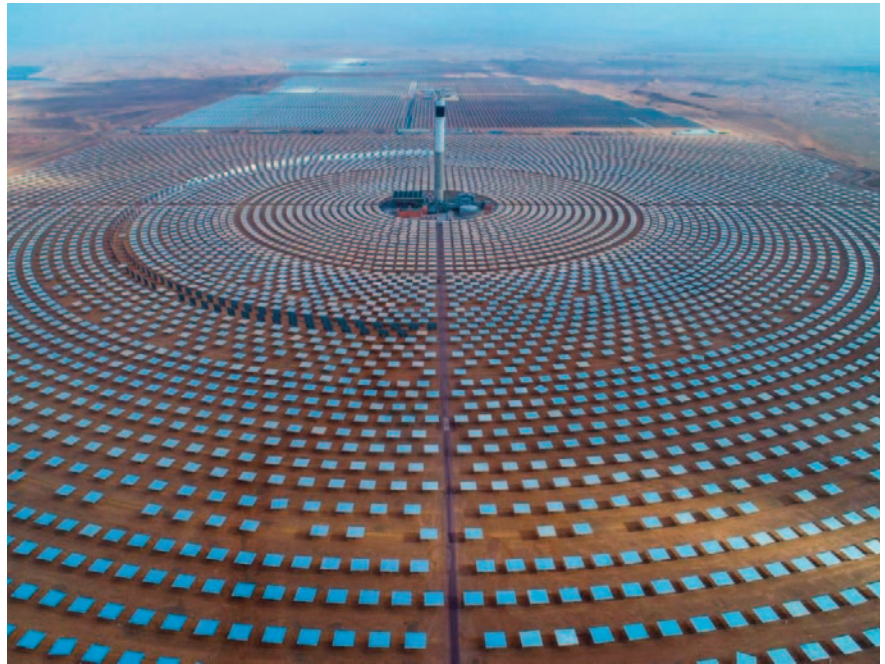
Noor Complex Solar Power Plant is located in the Sahara Desert and it is the world's largest concentrated solar power plant. The Solar Plant capacity is of 580 megawatts
