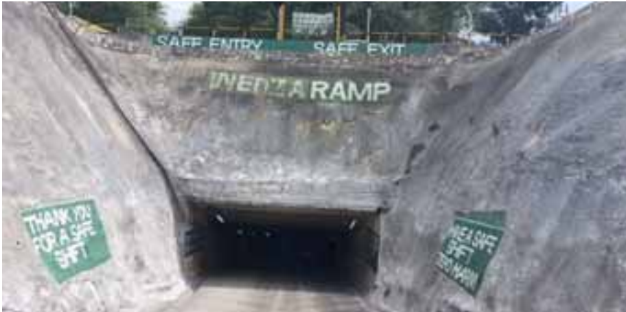
Wedza ramp at Mimosa Mining Company
