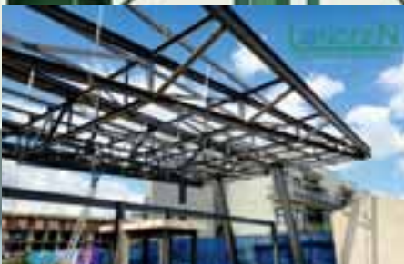
Rigging/ Erection of Steel Structures
