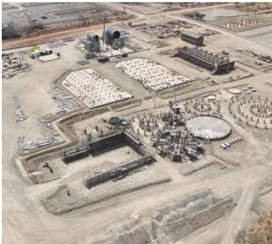
One of Zimbabwe's newest projects – Karo Platinum project in Ngezi
